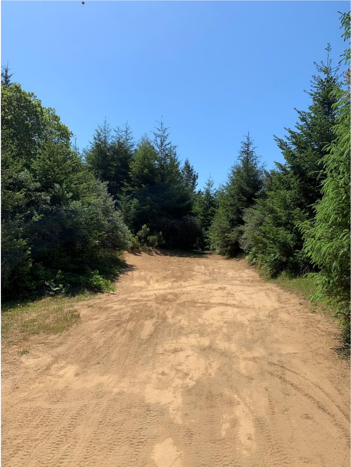
Figure 3 Unrocked Seasonal Haul Road on MCF
